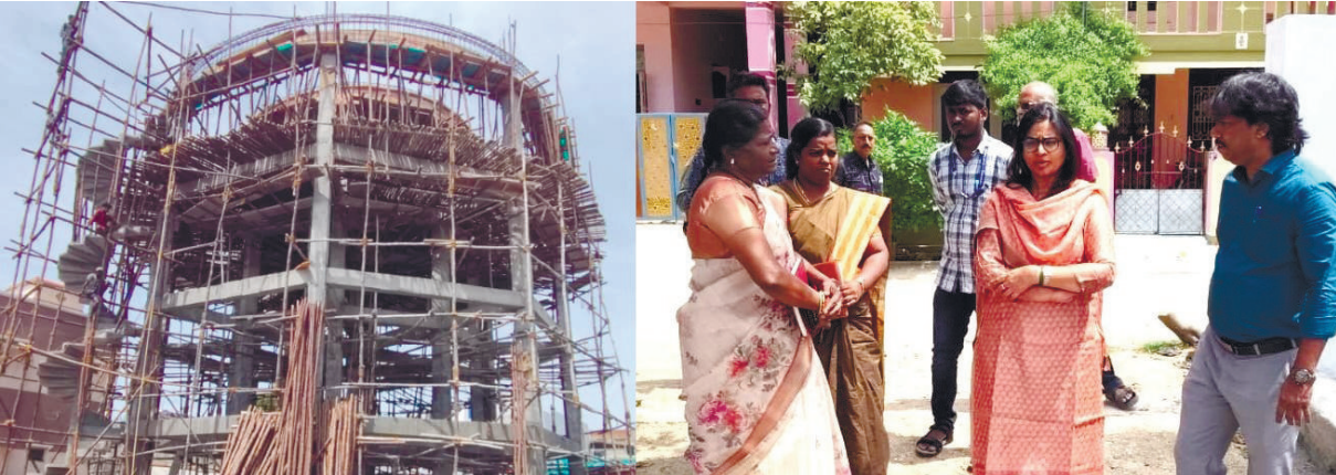
Ranipet Collector N. Priya Ravichandran inspected the Rs 21.24 crore drinking water improvement works being carried out under the AMRUT 2.0 scheme at Seven House in Arakkonam municipality.
